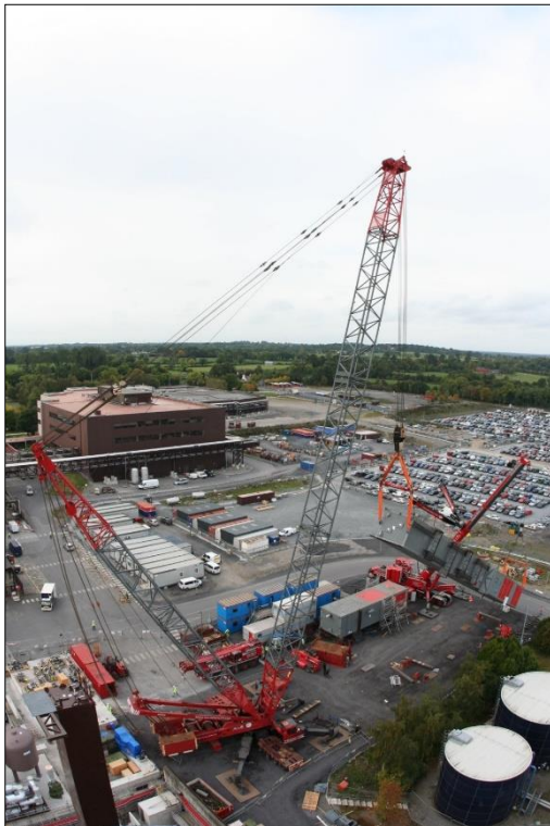
Figure 3-7: 1200 T Crane Example 2
