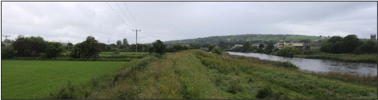
Figure 14-8: On bank of River Foyle, off site
